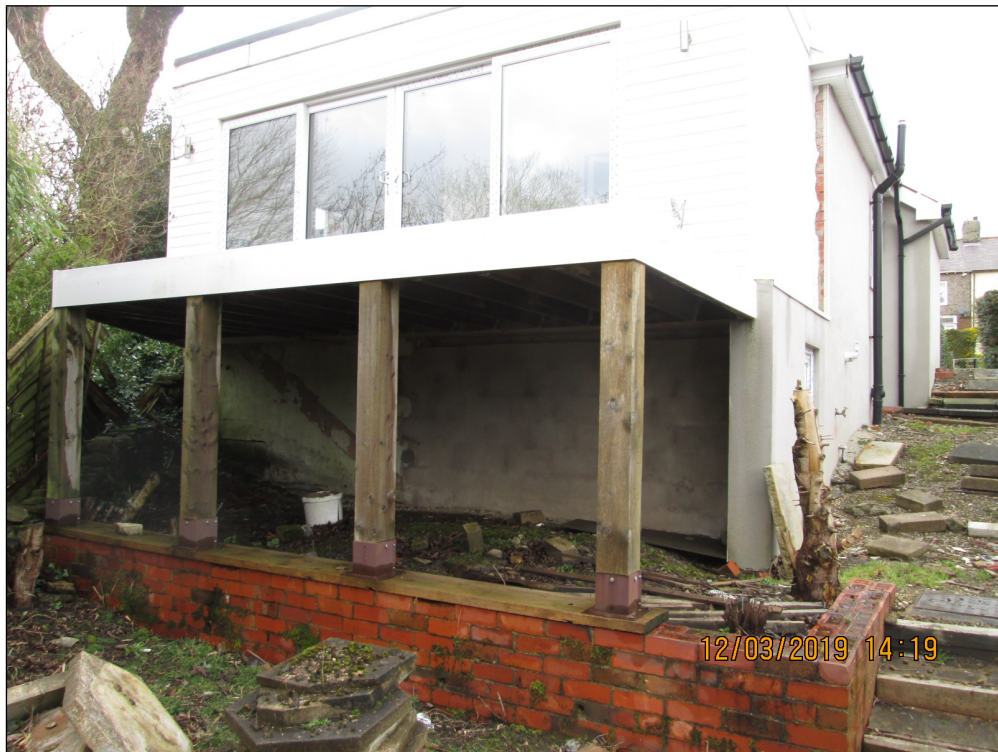
Raised platform for balcony
